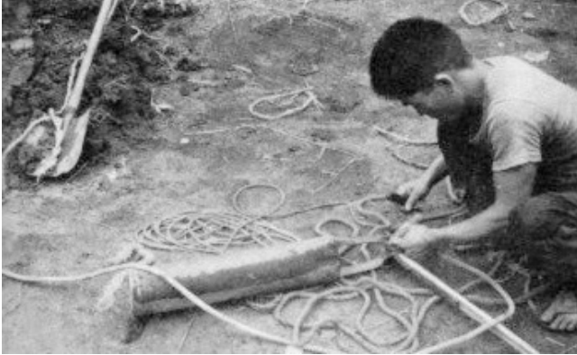
Phot. 6 Bits at the tips of Kazusabori well-boring tools
