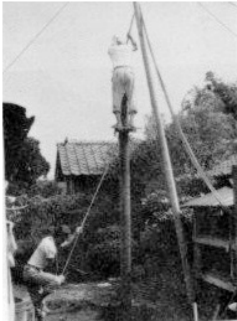
Phot. 5 Simple kazuabari well-boring method
